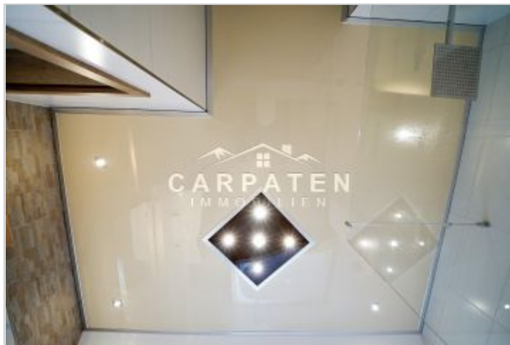
LED-Spots Badezimmer DG
